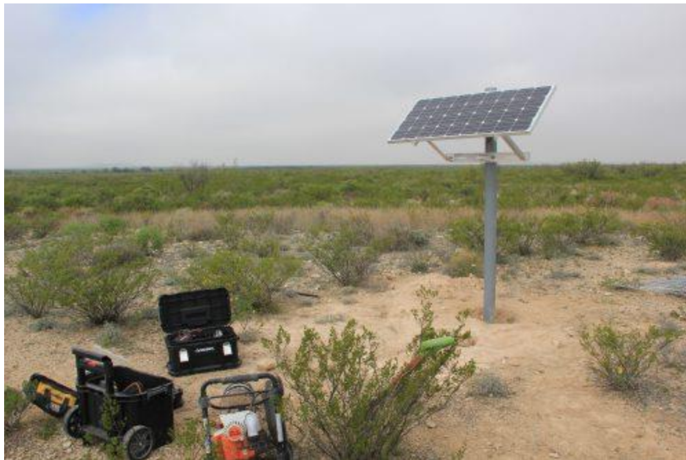
A TexNet seismic monitor being installed on ranch land in Pecos County. (Bayla Metzger)
